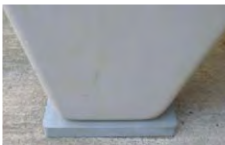
Machinery and tank levelling
