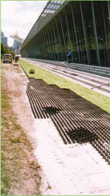
Melbourne Exhibition Centre during installation
