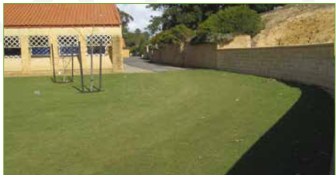
Service vehicle access, installed using Grassrings turf-reinforcement
