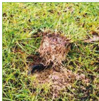
Note how the grass roots develop into the porous base course
